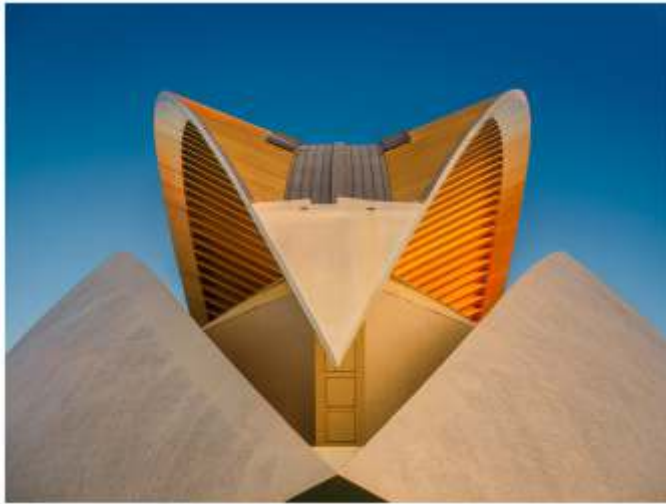
Salon Mention PDF BARRY DILLON, Ireland, Opera House Rooftop Valencia
